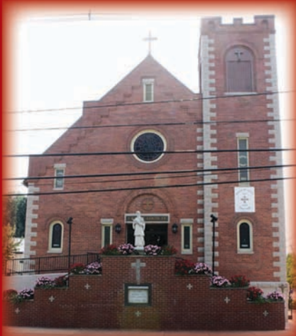
A complete rewiring of St. Louis Church, Gallipolis
